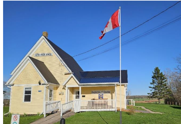
Riverview Community Centre (the “Centre”)
